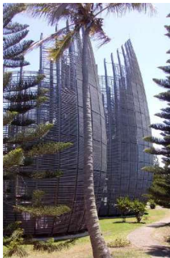
Glued laminated framework, Jean-Marie Tjibaou Cultural Centre - Nouméa, New Caledonia (picture J. Gérard).
